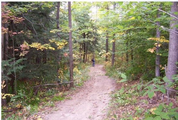
This section of trail is nearly finished being brushed and cleared.
